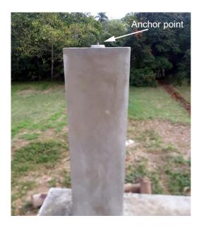
Figure 7. Concrete pillar with a platform for a GNSS antenna mounting.
